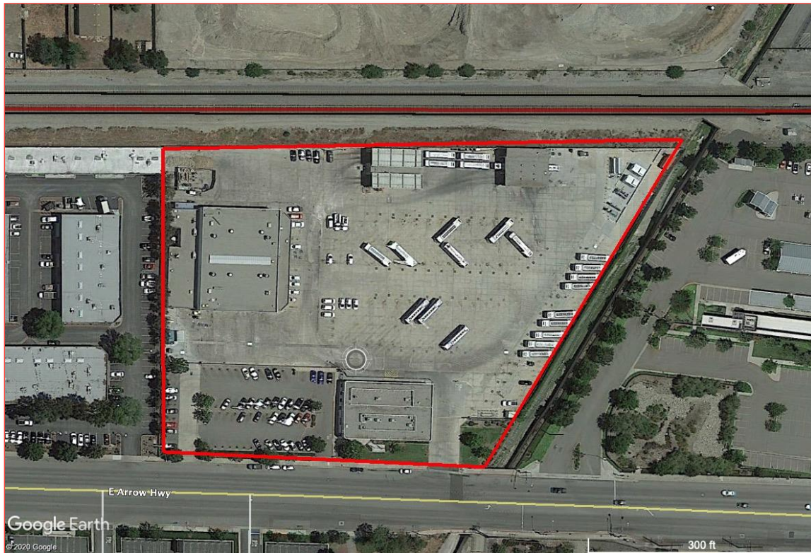
Figure 5-2. West Valley Division - Existing Conditions
