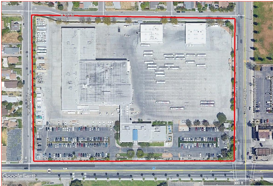
Figure 5-5. East Valley Division - Existing Conditions
